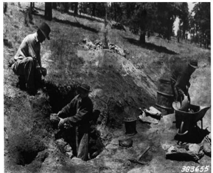
CCC workers receiving on-the-job instruction as they build a culvert in a road in the Apache-Sitgreaves National Forest, Arizona.
