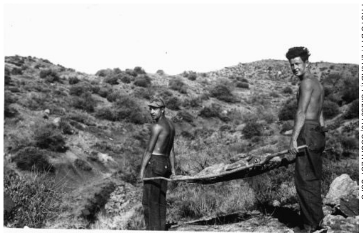
CCC workers carrying rocks for erosion check dams, Tonto National Forest, Arizona
